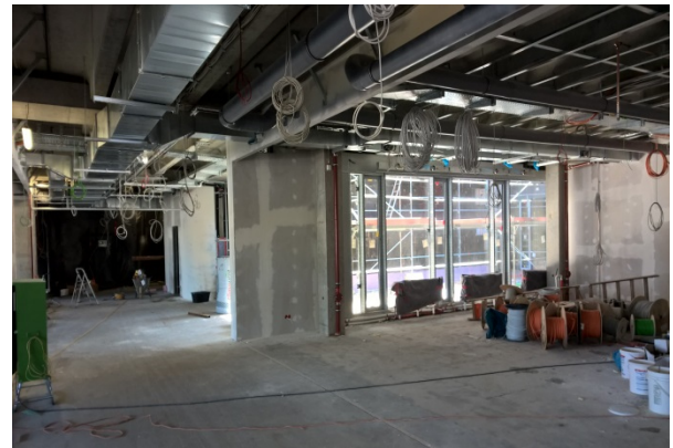
Rohinstallation Elektro
